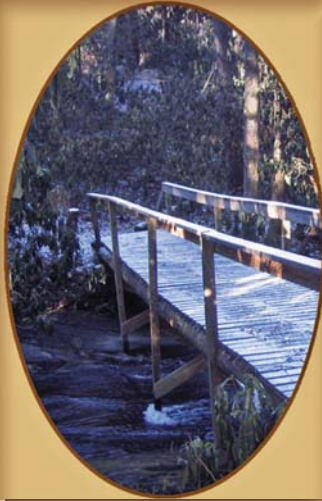
Mill Creek Bridge
